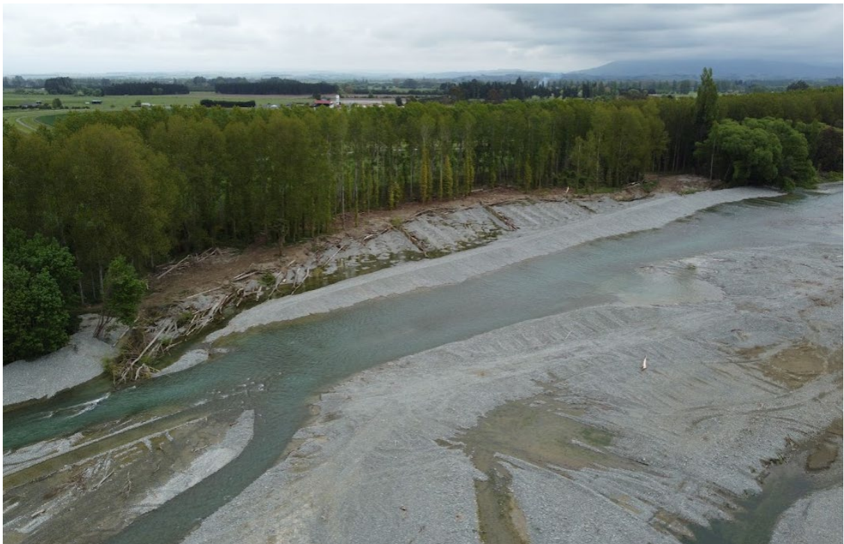
Figure 2-3: Anchored tree edge protection replacement repair where erosion was within 30m of stopbank edge. Orari River at Racecourse. Job 23715.
