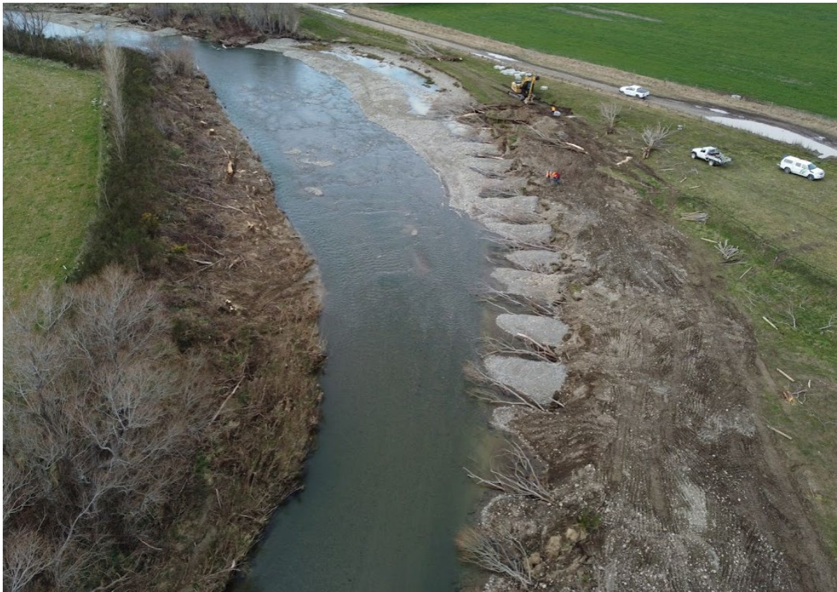
Figure 2-4: Anchored Tree Protection installation underway. Bowyers Stream. Job 23871.
