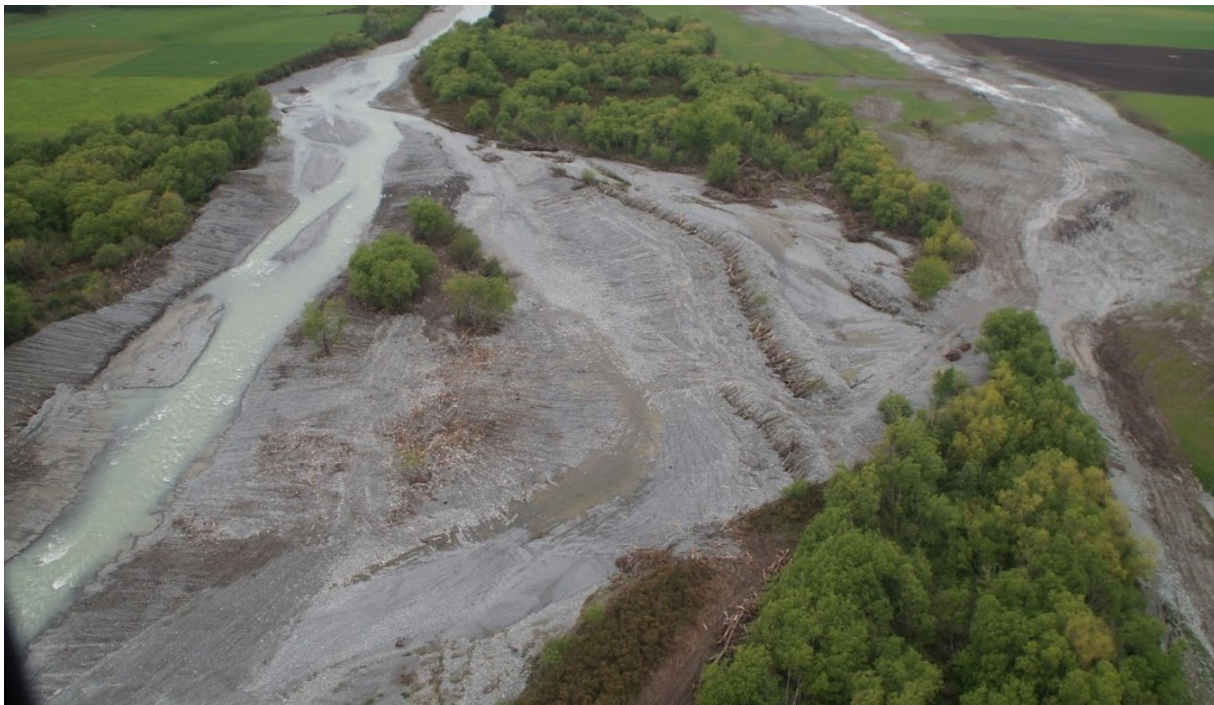
Figure 2-5: Completed stream diversion, buried tree line, deflection bunds. South Ashburton River. Jobs 23632 & 23633.
