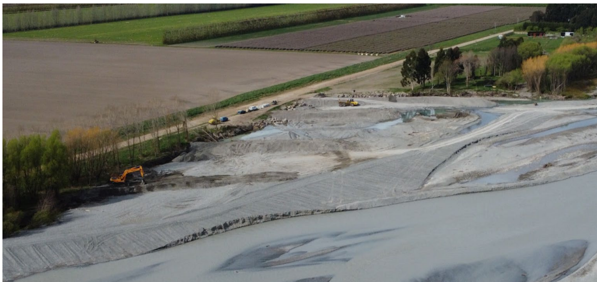
Figure 2-1: Erosion Protection Bunds under construction with tree edge replacement (Anchored Tree Protection) yet to start. Ashburton River. Job 23545.
