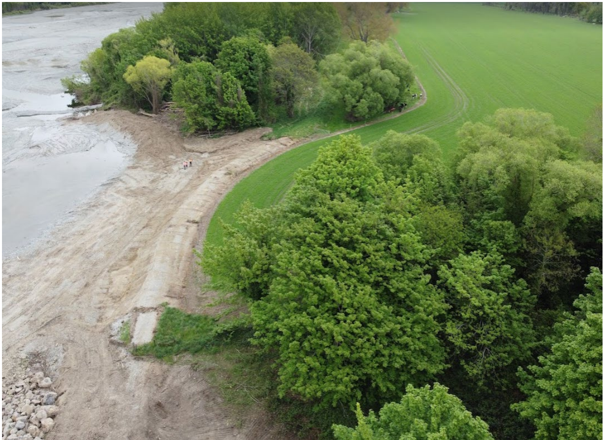
Figure 2-2: Stopbank repair underway with tree edge replacement yet to start. Orari River at Railway Bridge. Job 23718.
