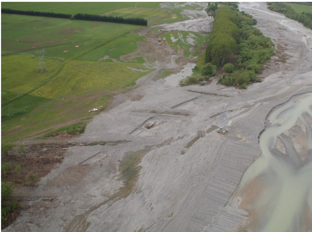
Figure 2-7: Completed Anchored Tree Protection Groynes. South Ashburton River. Job 23590.
