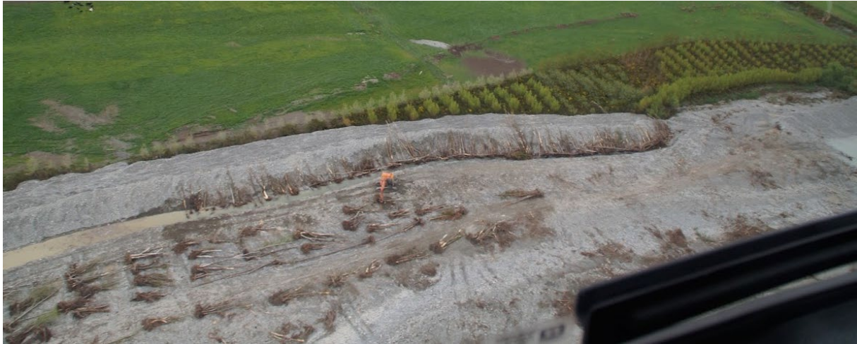
Figure 2-6: Buried Tree line during installation. South Ashburton River. Job 23628.
